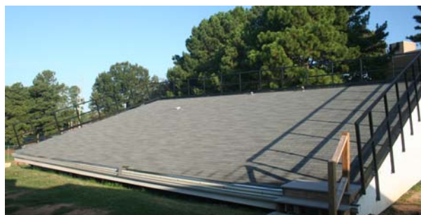
28' x 48' 4/12 pitch training roof for photovoltaics and solar thermal hands-on training
