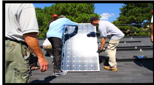
28' x 48' 4/12 pitch training roof for photovoltaics and solar thermal hands-on training
