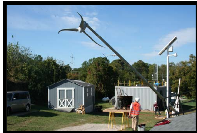
A Skystream 3.7 on a 60 foot tower being lowered for training purposes.
