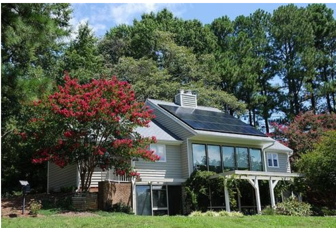
The NCSU Solar House on N.C. State's Campus serves as a demonstration of renewable energy and energy efficiency
